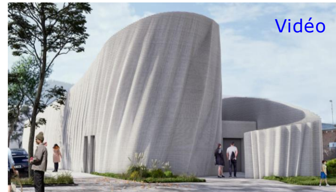
Wave House data center (Heidelberg, 2024) PERI 3D Construction, 600 m 2 en 140h
