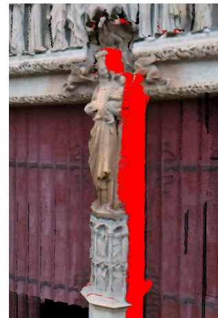
Figure 9: The south portal point cloud colorized. The points re-colored in red are invisible from the digital image pose
